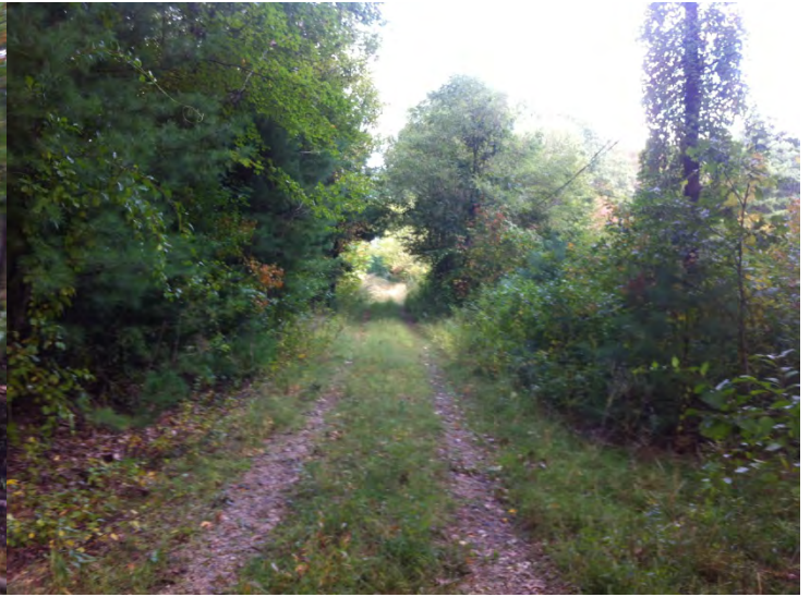
View north of the rail trail from culvert #2
