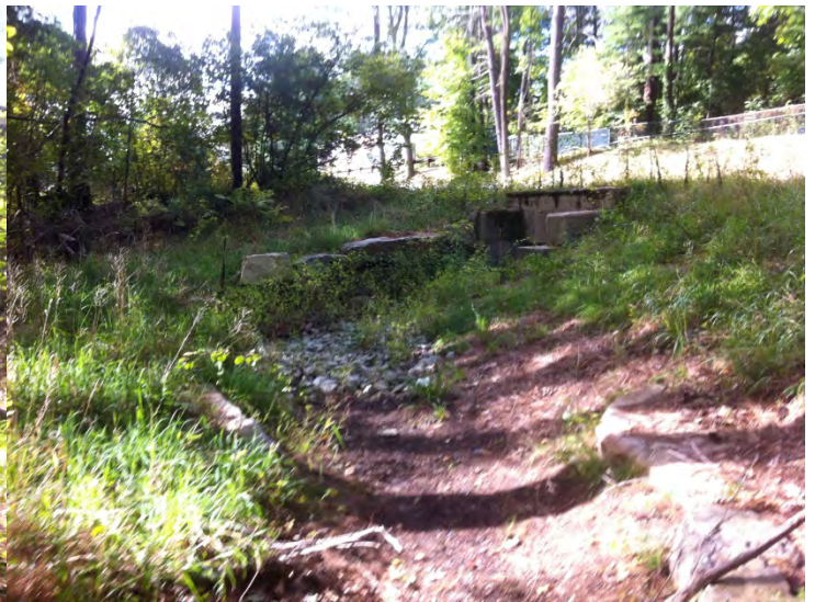
View south of culvert #2
