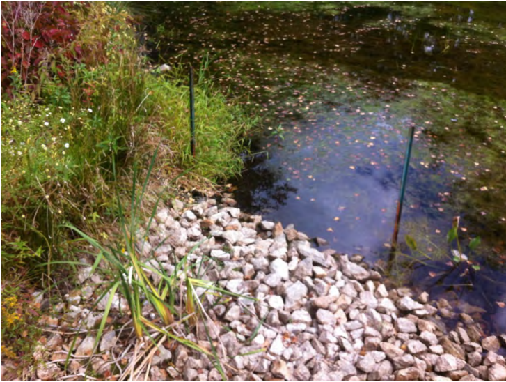
View of culvert #1 inlet to the vernal pool
