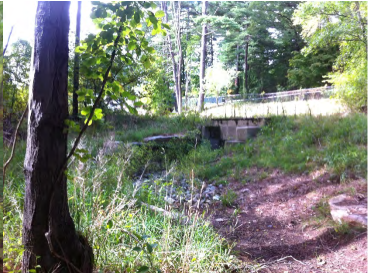
View south to culvert #2
