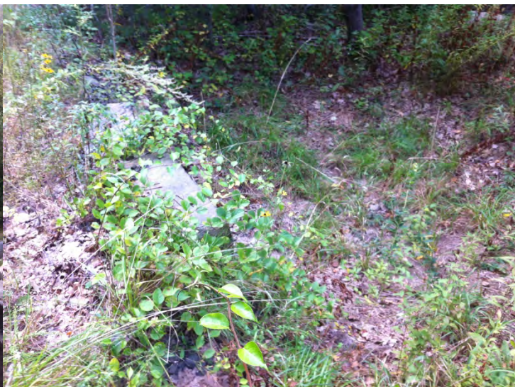
View of culvert #3 just south of the access way.
