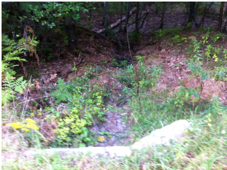
View east of culvert #3
